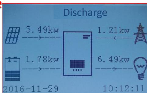
When the sum of the power produced by the photovoltaic system and supplied by the battery is less than that required by the loads, the missing energy will be taken from the grid.
